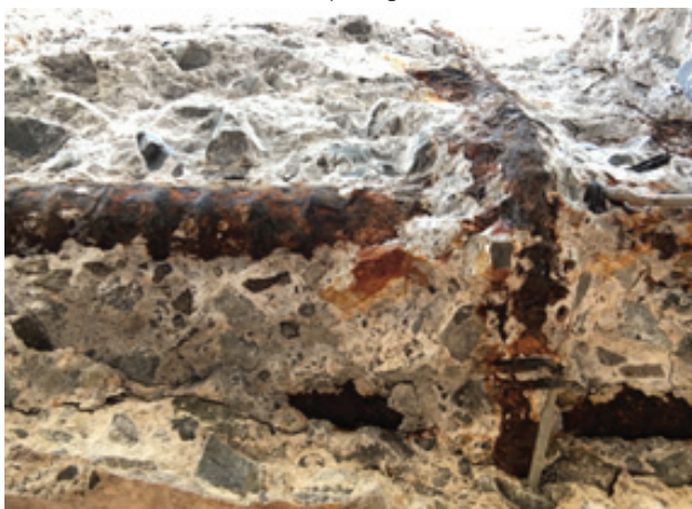
Bent corner of a stirrups
