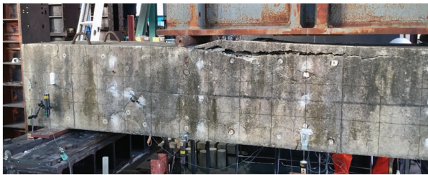
Figure 8 The appearance of the beam after the loading test
