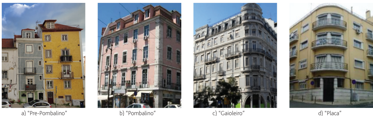
Figure 1 Pre-code masonry buildings in MAL
