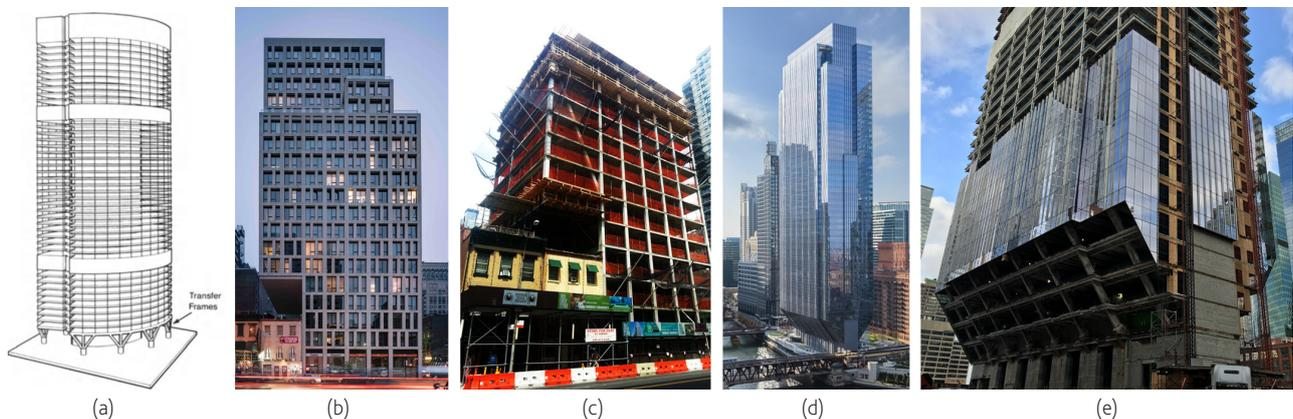
**Figure 6** (a) Structural system of the Grosvenor Place, Sydney, Australia; (b) 160 East 22nd Street Building, Manhattan, New York, USA; (c) Inclined column view during construction of the 160 East 22nd Street Building; (d) 150 North Riverside Plaza, Chicago, USA; (e) Inclined columns of the 150 North Riverside Plaza
