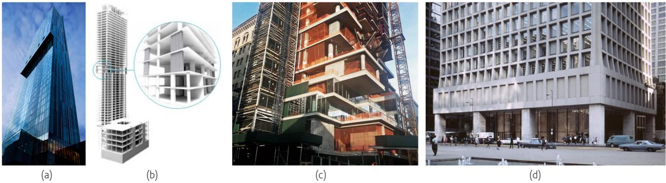
**Figure 7** (a) Beetham Tower, Manchester, UK; (b) Walking column system at the Beetham Tower; (c) Walking column at the 56 Leonard, Manhattan, New York, USA; (d) Deep beam in the Brunswick Building, Chicago, USA
