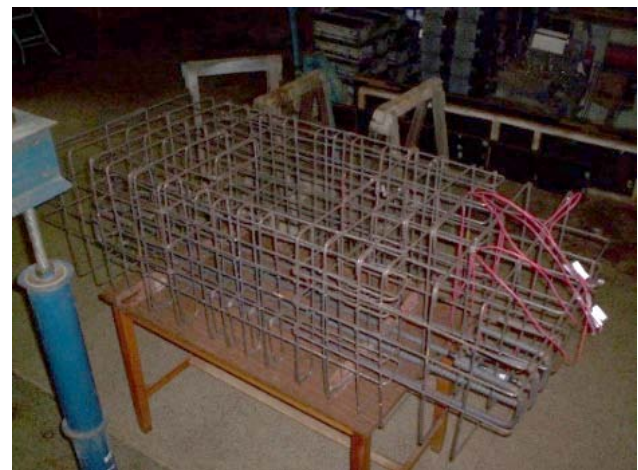
Figure 5 Arrangements of the pile caps' steel bars
