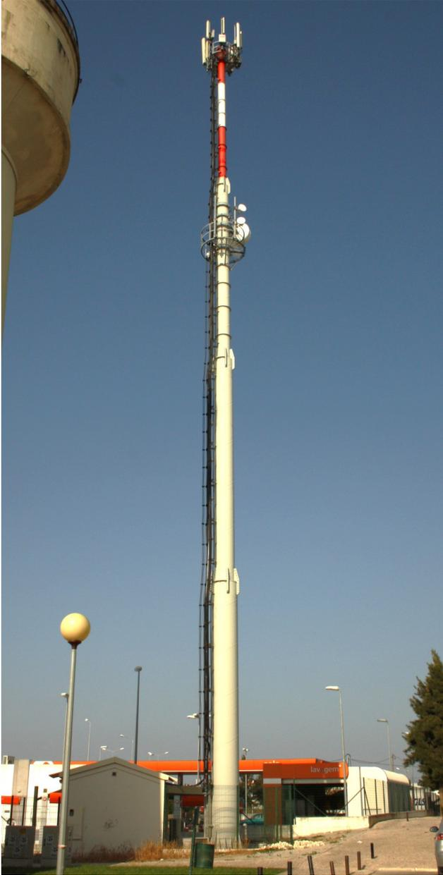
a) Monopole with a circular cross-section
