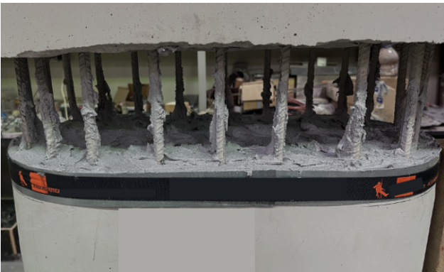
(a) preenchimento com SikaDur-30
